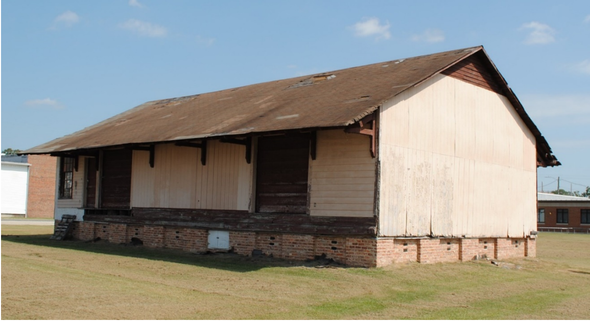
Figure 8 Erwin Depot Building
