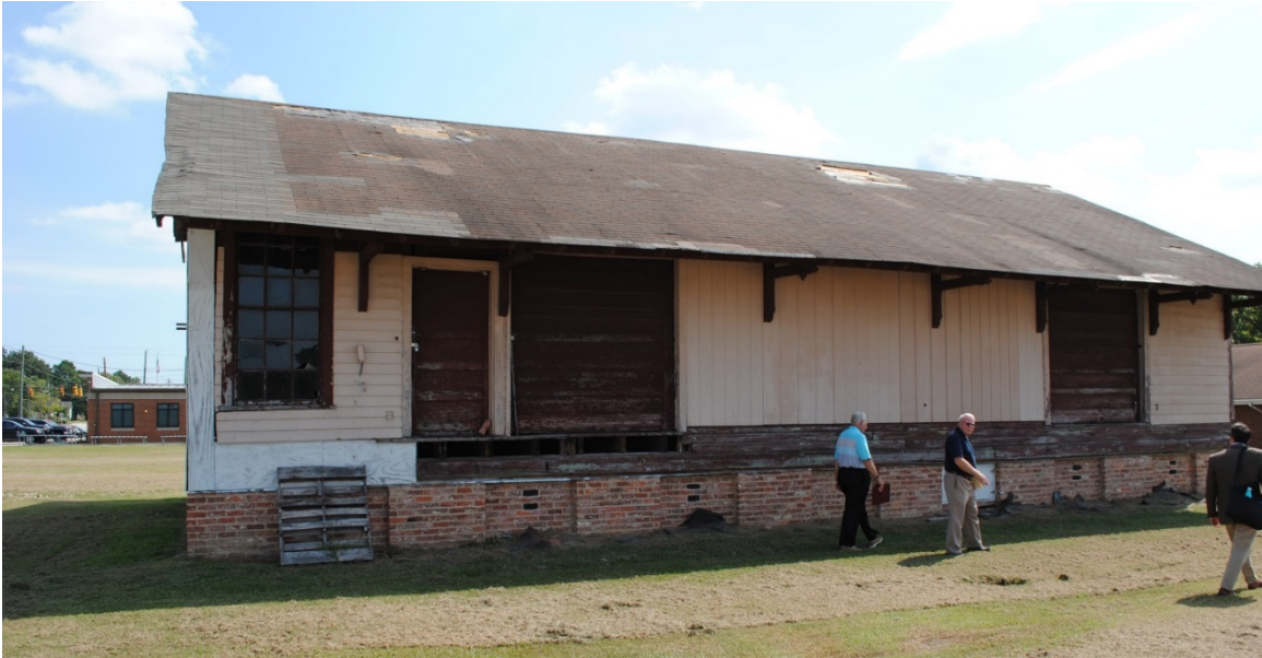
Figure 7 Erwin Depot Building
