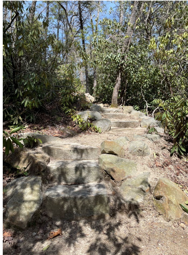
Finished steps on Grassy Creek Falls Trail.
