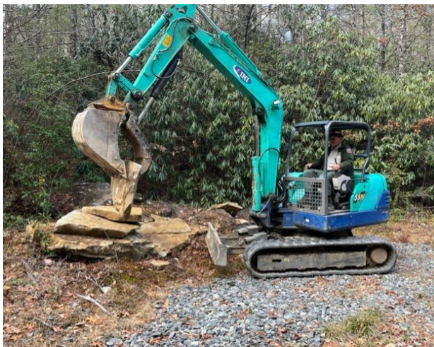
DSRF ranger lifts large rocks for use in a stream crossing.
