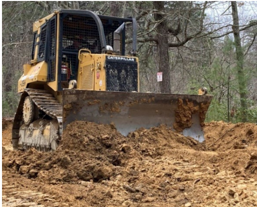
DSRF staff grading for the overflow parking area.
