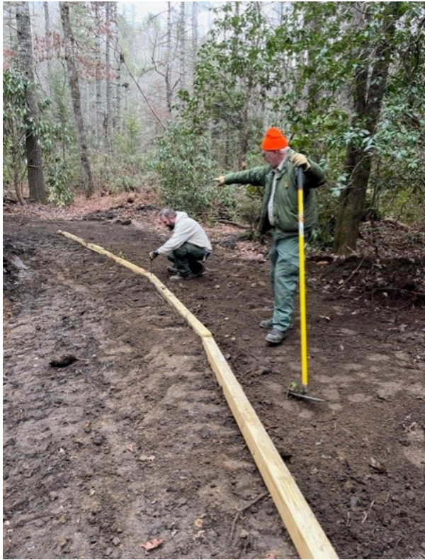
Two rangers building a "turnpike" for a persistent, muddy section of trail.
