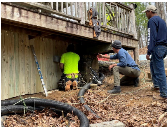
Contractors enclosing the lower level of the law enforcement cabin.
