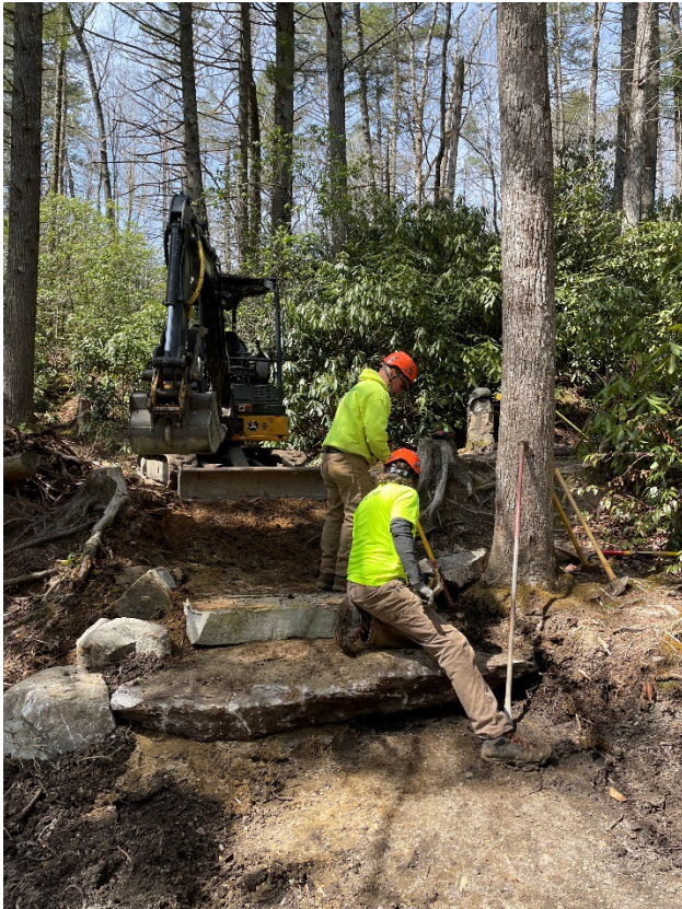
Trail contractor installing steps along Grassy Creek Falls Trail.
