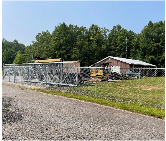
Fencing around the maintenance facility improves security and safety.
