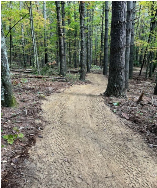
Hooker Creek Trail repairs completed.
