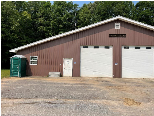
The DSRF maintenance facility is scheduled for renovation.
