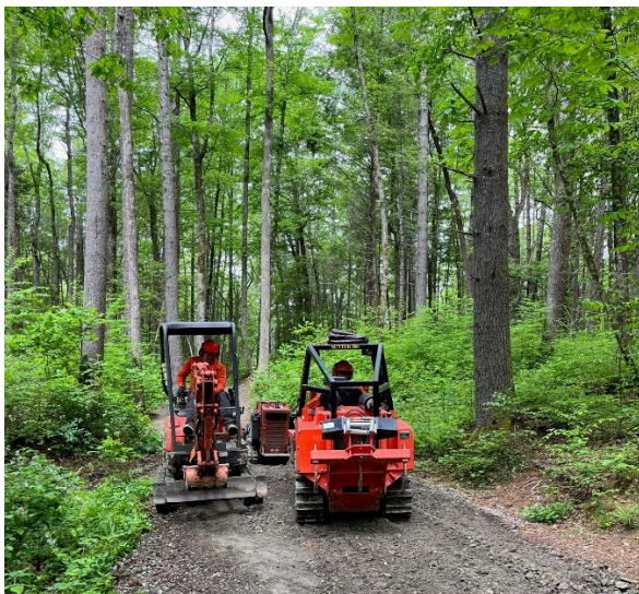
A trail contractor makes improvements to Hooker Falls Trail.
