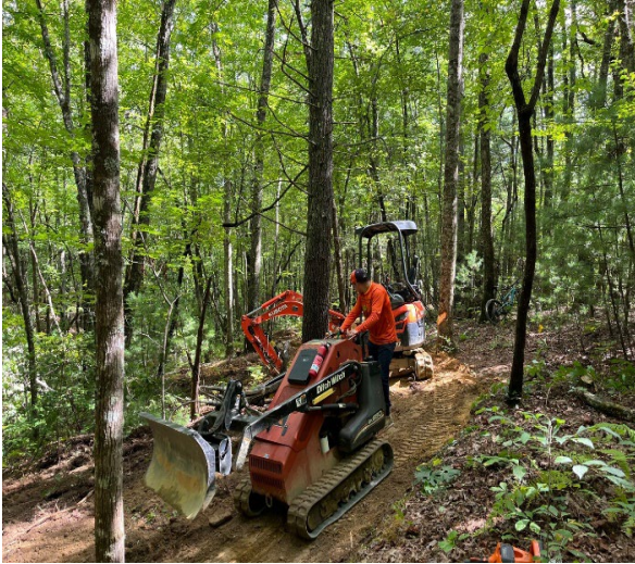
Contractors working on Jim Branch Trail.
