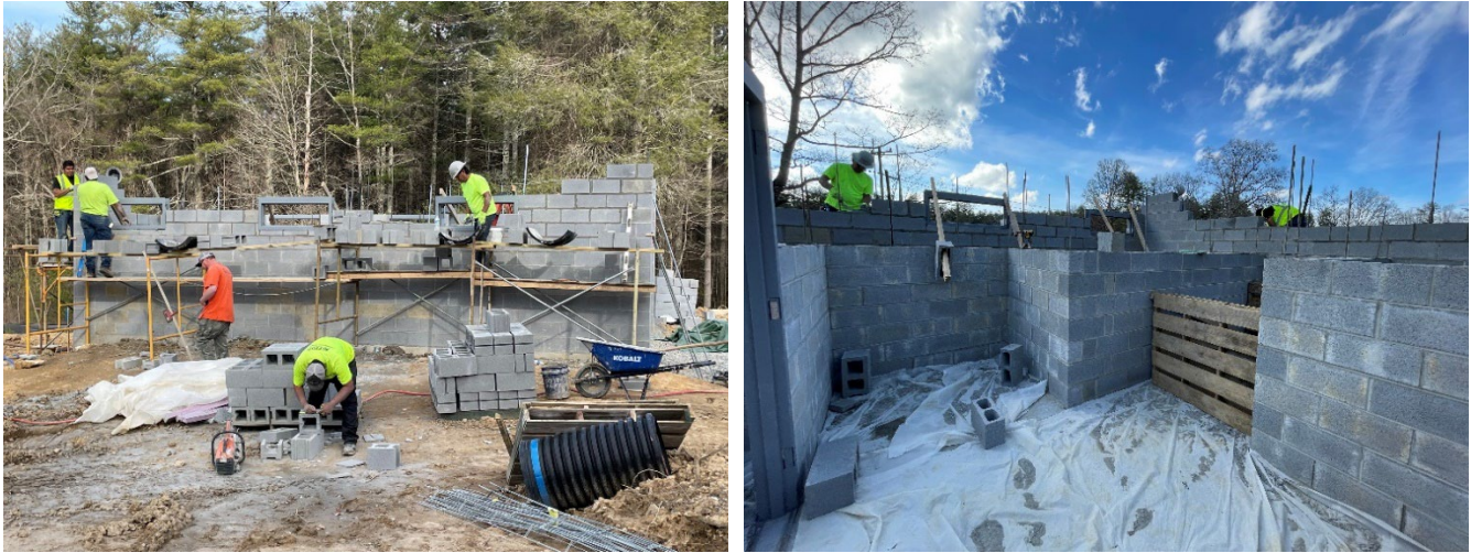
Work under way on the Guion Farm Access Area restroom.
