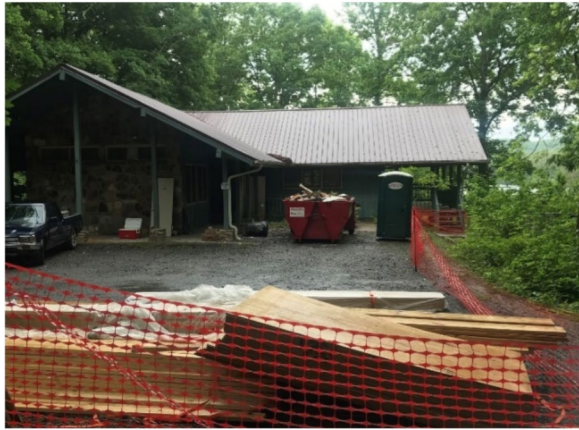
Renovation progress at Lake Julia office
