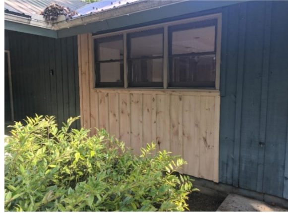
Exterior repairs to Lake Julia office
