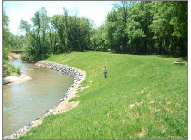
Stream restoration (after), Caldwell County
