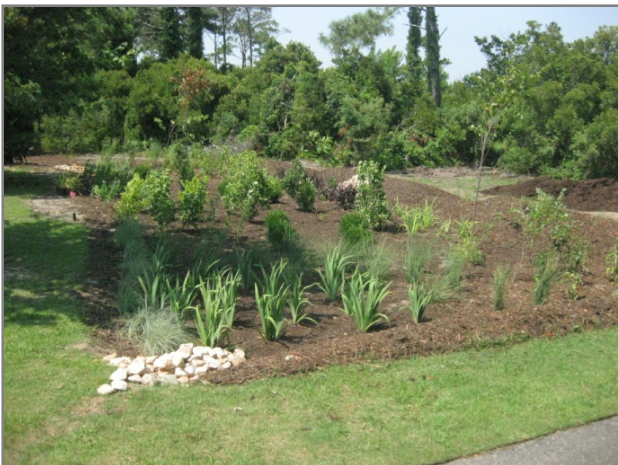
Bioretention area, Dare County
