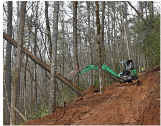
Trail construction near Hooker Falls
